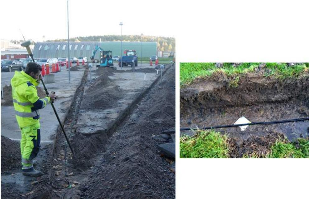
*Figure 10. Permanent installation of electrodes for a DCIP monitoring experiment. Alingsås, Sweden.*
