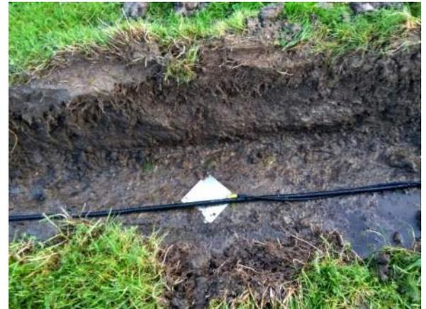
*Figure 2. Monitoring installation of the stainless-steel plate electrodes. The electrodes and the cables are buried 30 cm under the surface to ensure a permanent installation.*
